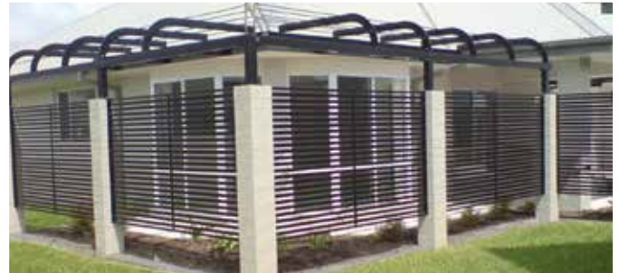
Horizontal Slat Semi-Privacy screens to allow airflow, light and a courtyard barrier to this retirement village
