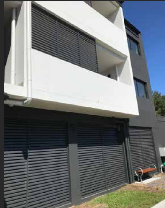
Carpark and balcony privacy louvres
