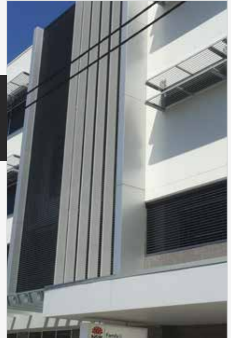
Service NSW - Mayfield Vertical RHS Battens with Grid Screening and Twin Sunhoods
